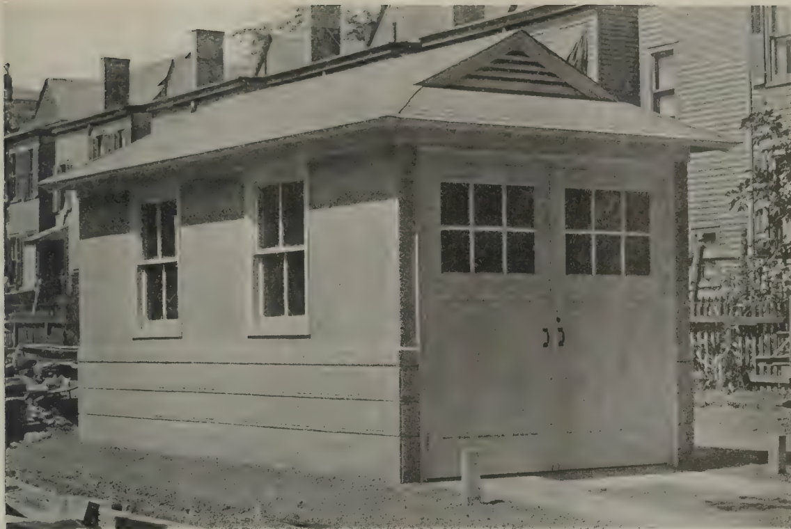
The Completed Garage
